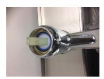
4 if water was leaking around the brass nut then try tightening up before changing as the nut may be loose. If water was coming around the square shaft then remove nut and change cartride. Do not over tighten. Once nut is reinstalled turn water back on and check for leaks incase the nut needs further tightning.
